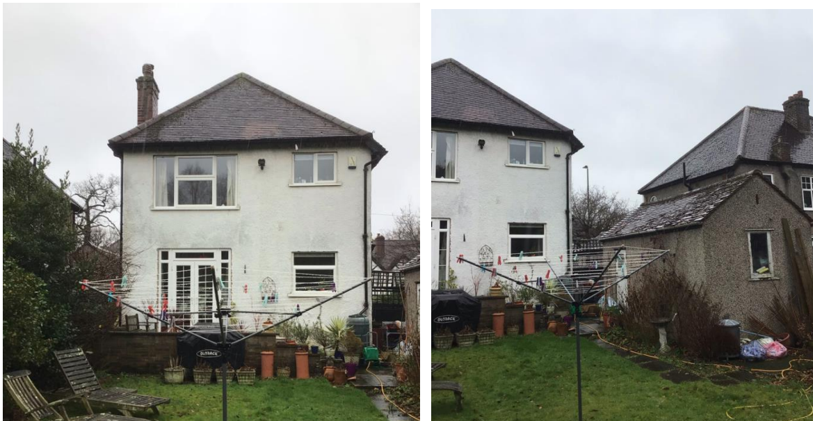
Figure 7: Photograph of Rear Elevation
